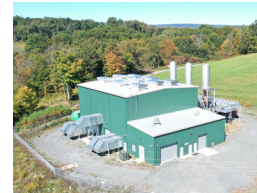
Wolf Run Energy LLC Wilmont Township Bradford County, PA COD: June 2019
